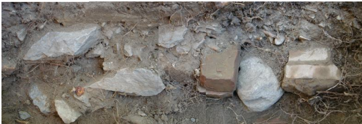
Figure 7: A partial view of the brick wall, Feature 5
