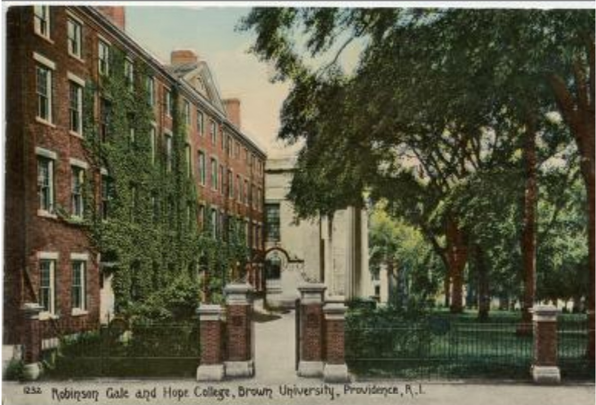
FIGURE 2.14. Robinson Gate and Hope College. Photograph facing south, 1908-1911. Textual records indicate that ivies were growing on Hope as early as 1903 and that by 1908 half covered the building. In this figure, there is more ivy on the walls of the edifice than shown in Figure 2.12, but less than in Figure 2.14.
